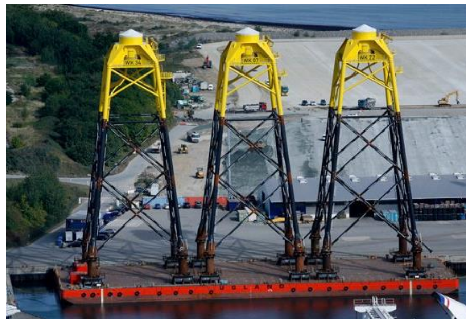
Figure 10 Four-legged jackets en-route to the Wikingen wind farm. (Source: Iberdrola).
