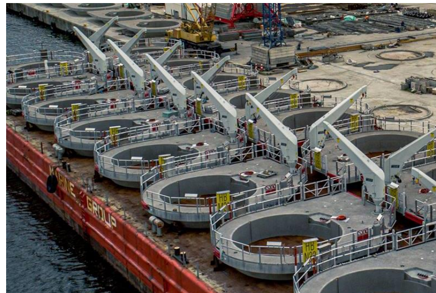
Figure 7 Concrete work platforms. (Source: Aarsleff).
