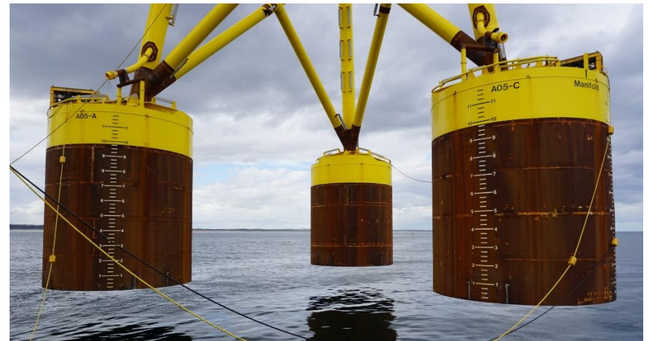
Figure 14 Jacket with suction anchors being installed at Borkum Riffgrund. (Source: Framo).
