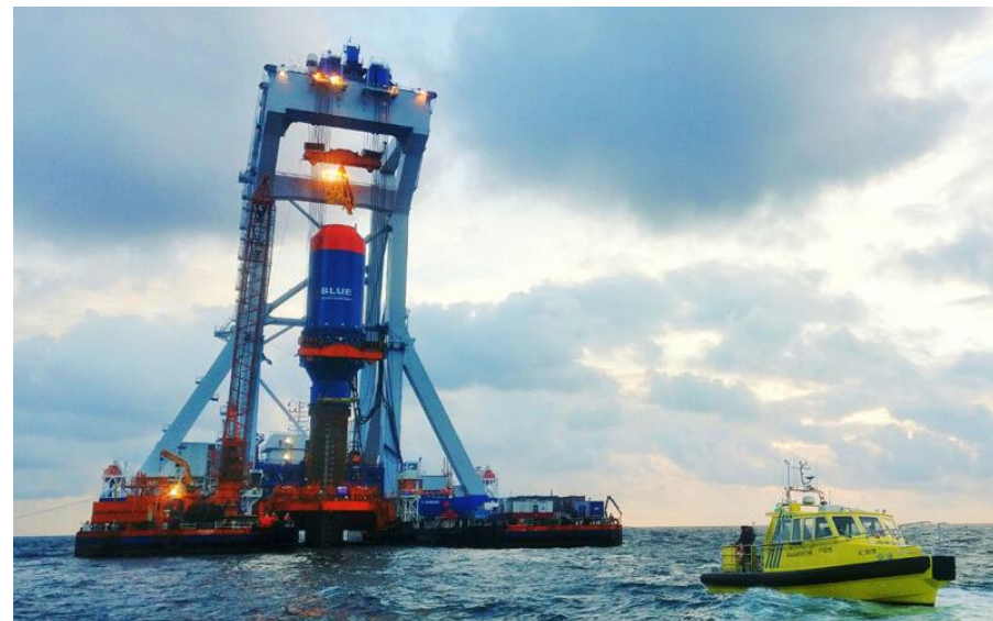
Figure 45 BLUE piling under test. (Source: IQIP).
