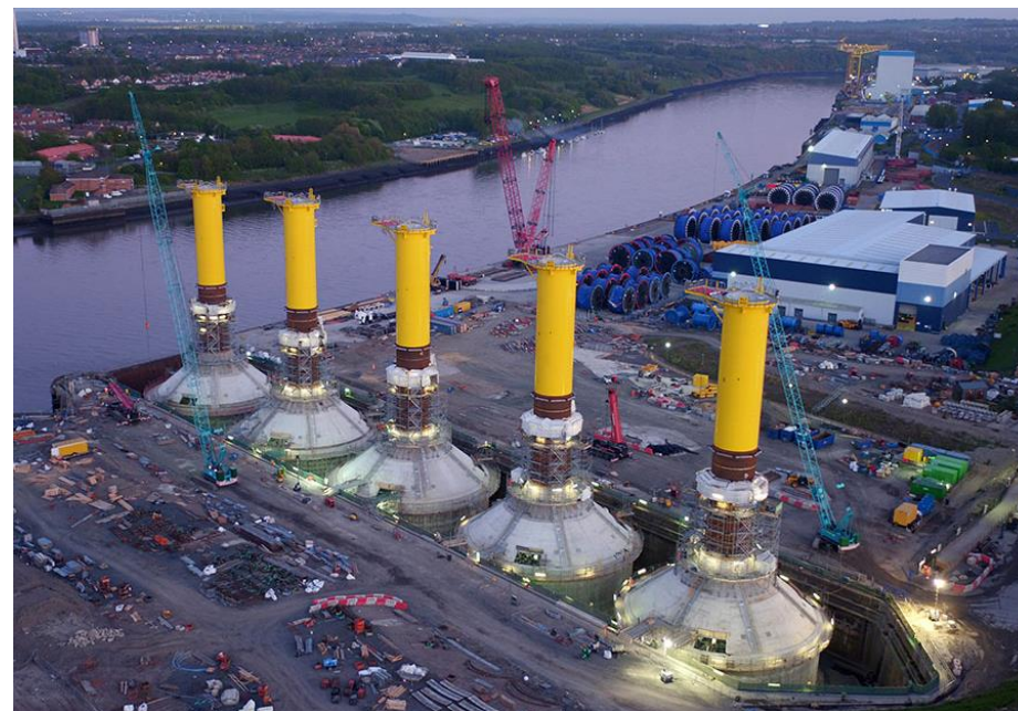
Figure 15 BAM Nuttall concrete GBFs for Blyth windfarm, using steel shafts. (Source: BAM).
