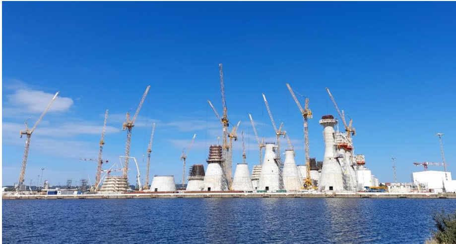
Figure 17 Industrialised construction of GBFs by Bouygues Travaux Publics at Le Havre for Fécamp. (Source: Bouygues).
