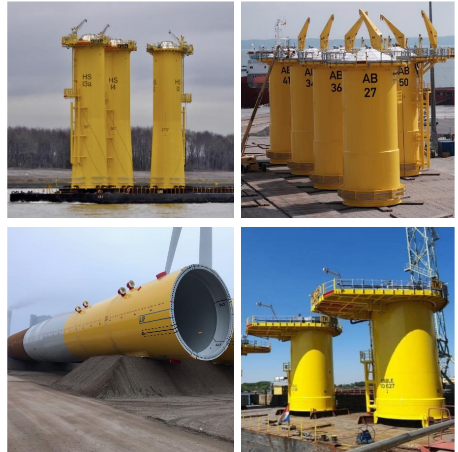
Figure 6 Examples of MP/TP variants. Clockwise from top left: grouted (Hohe See, EnBW), conventional bolted (Arkona, E.ON), compact bolted (Triton Knoll, RWE innogy), and “TP-less” monopile (Hollandse Kust Zuid 1-4, Vattenfall).
