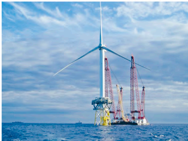
Figure 3 The Scottish offshore Beatrice Demonstrator was the first in the world to use large 5MW turbines and deep water jacket foundation technology.
