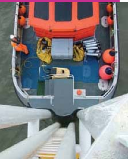
A specially designed access system from a work boat to a turbine.
