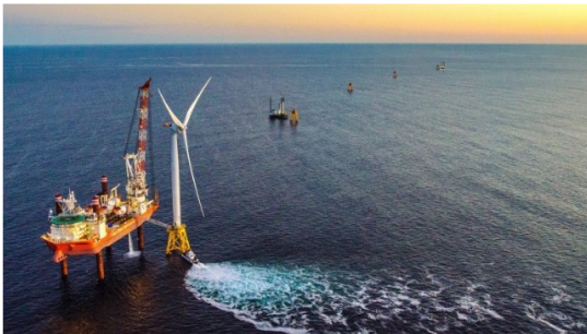
Block Island windfarm installation
