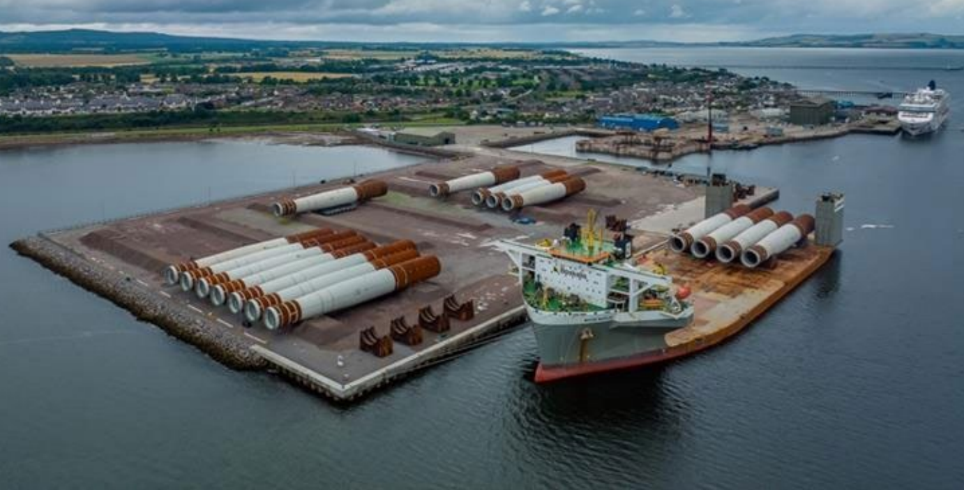
Port of Cromarty Firth supported monopile installation at Ocean Winds 882 MW Moray West project (Credit: Sarens)
